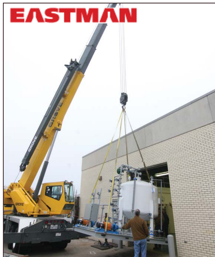
(Above) A crane hoists the new industrial-sized "flow loop" into the M. Kenneth Whitten Applied Technology Center. The device will give students hands-on training for a career in process technology.
